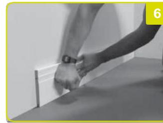
**5.** Apply sinuous and continuous lines of Heavy Duty Adhesive according to the size of your profile:
