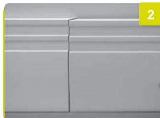
**1.** When installing Santa Luzia's bases and casings on a long wall, you can join several bars together. To do this, cut the ends of the bars at a 45° angle (by adjusting the bevel), using an electric mitre saw with a 96 teeth blade and 12 inch diameter.
