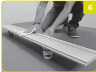
**7 and 8.** Apply two parallel lines of Glue or Heavy Duty Adhesive on the backside of the bar. For bar over 5-7/8" (15cm) in width/height, apply at least 3 lines of Heavy Duty Adhesive. Then, place the bar where it will be applied and with your hands, make sure it connects to the T-Brackets you previously applied on the wall. Wipe off excess Glue or Heavy Duty Adhesive from the profile after installation.
