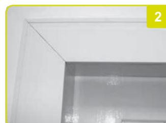
**1** Make straight cuts with the miter saw, at a 45° angle (adjusting the mitre), with the cases flat (horizontal position).
