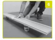
NOTE :In places where the wall cannot be drilled (for example, when there is a hydraulic network) a small piece of double-sided tape can be used every 15-¾" (40 cm) with Heavy Duty Adhesive, avoiding drilling.
